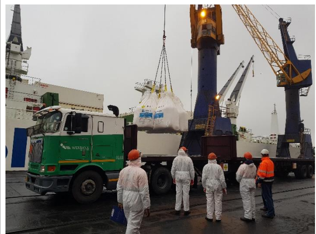
6. Shore cranes loading bags from a platform onto a truck.
