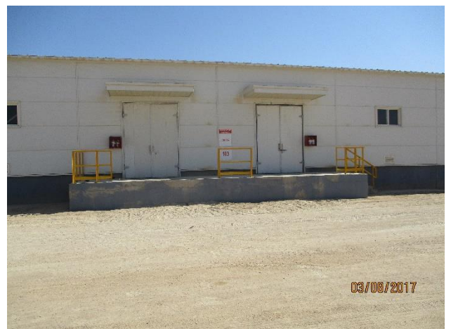
12. Warehouse used for the storage of AN.
