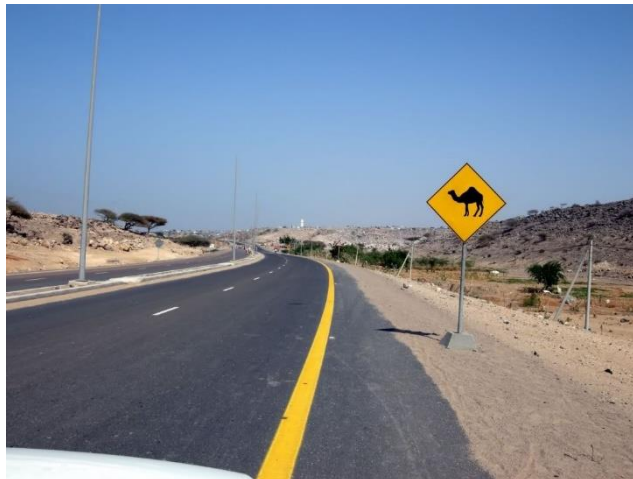
Figure 9 – A surfaced road in Djibouti
