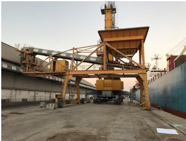
11. Crane, bulk hopper and conveyor in position ahead of discharge.
