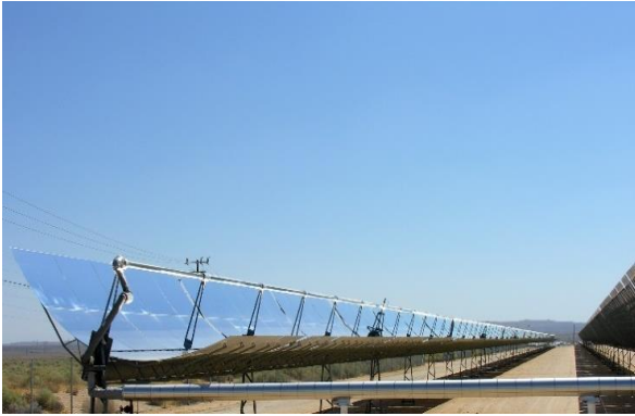
Figure 14. Parabolic trough solar thermal collector.
